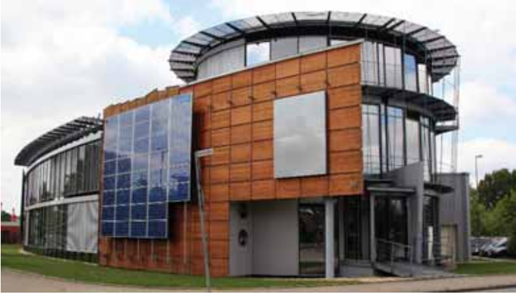
Many people remain wary about the viability of new 'green' technologies – whether they'll continue to work in the long-term and provide reasonable payback
