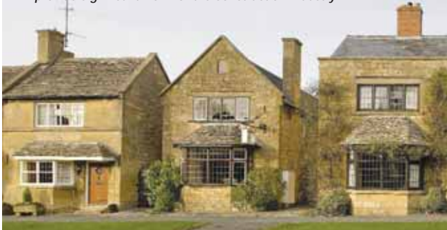
Reducing carbon emissions from existing housing stock will provide significant work for the construction industry
