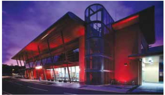
Willmott Dixon Turner's new A&E department at the West Wales General Hospital, Carmarthen
