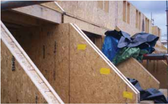
I-section joists used as structural timber studs
